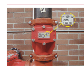
EXHIBIT L4.7 Check Valve Listed for 200 psi (13.8 bar). (Courtesy of JENSEN HUGHES, Inc.)
