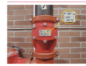
EXHIBIT L4.7 Check Valve Listed for 200 psi (13.8 bar). (Courtesy of JENSEN HUGHES, Inc.)
