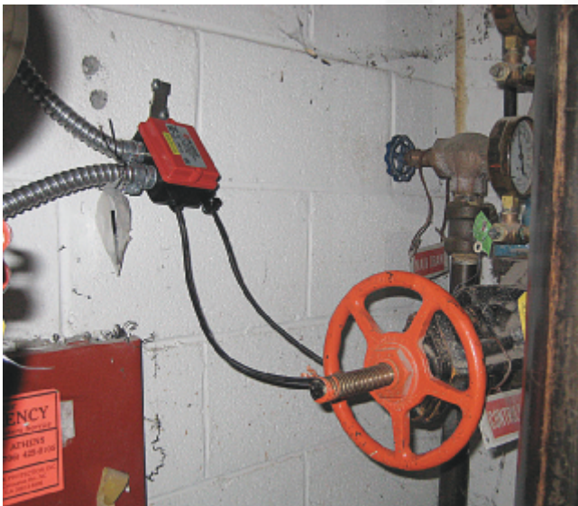
EXHIBIT 13.21 Valve Monitored by Wire Laced Through Handle.
