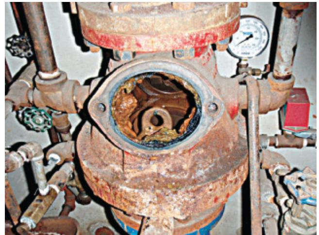
EXHIBIT 13.23 Interior Valve Corrosion. (Courtesy of Wayne Automatic Fire Sprinklers, Inc.)
