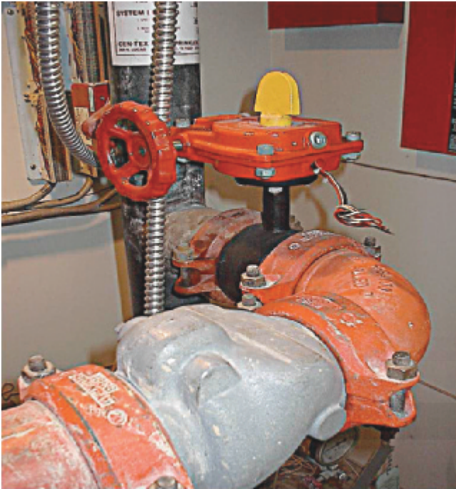
EXHIBIT 13.19 Butterfly Valve with Built-In Supervisory Switch (Not Wired).
