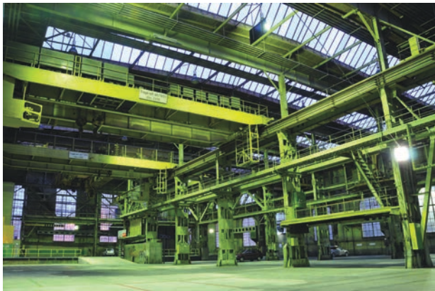
Figure 24. Overhead and side windows combined with electric lighting provide relatively uniform lighting in this space. The light colored floor reflects light to the underside of the large structures.
