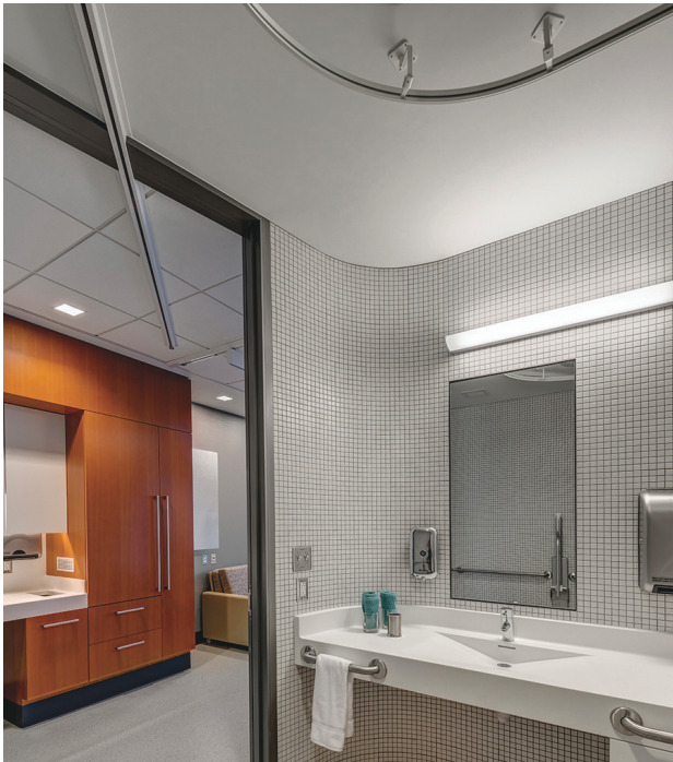
Figure 8-19. It is important that the ceiling lighting be coordinated with the location of bariatric lift tracks, which can run from patient room to bathroom to reduce the likelihood of falls during bathing and toileting. (Photo courtesy of Anton Grassl/ESTO)
