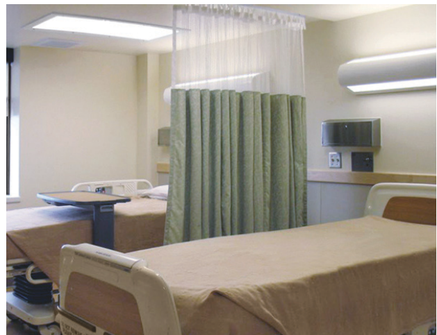
Figure 8-26. Behavioral health patient room utilizing tamper-proof security recessed lights and an anti-ligature wall-mounted luminaire for ambient and reading light. (Photo courtesy of Kenall)
