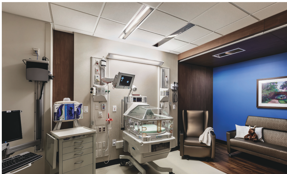
Figure 8-23. Indirect lighting is often used in neonatal intensive care units, minimizing the impact of glare on sensitive infants. (Photo courtesy of HDR; © 2013 balloggphoto.com)
