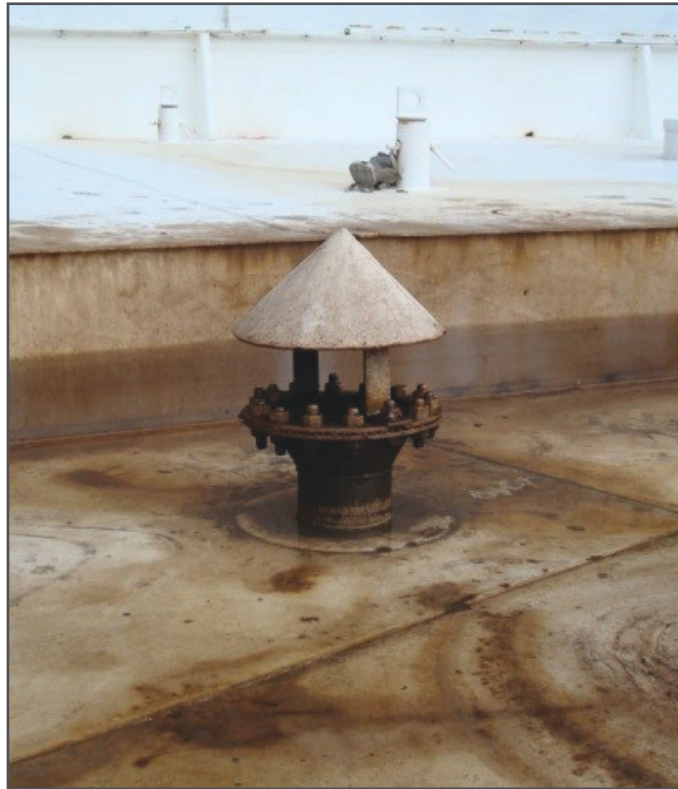
Figure 11-9 Typical emergency roof drain
