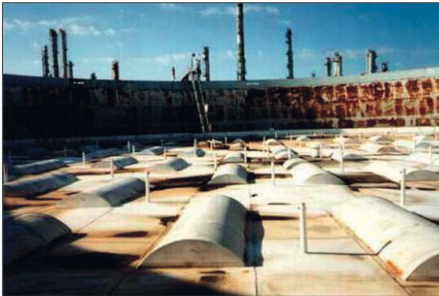
Figure 11-5 Example of buoy type radially reinforced roof
