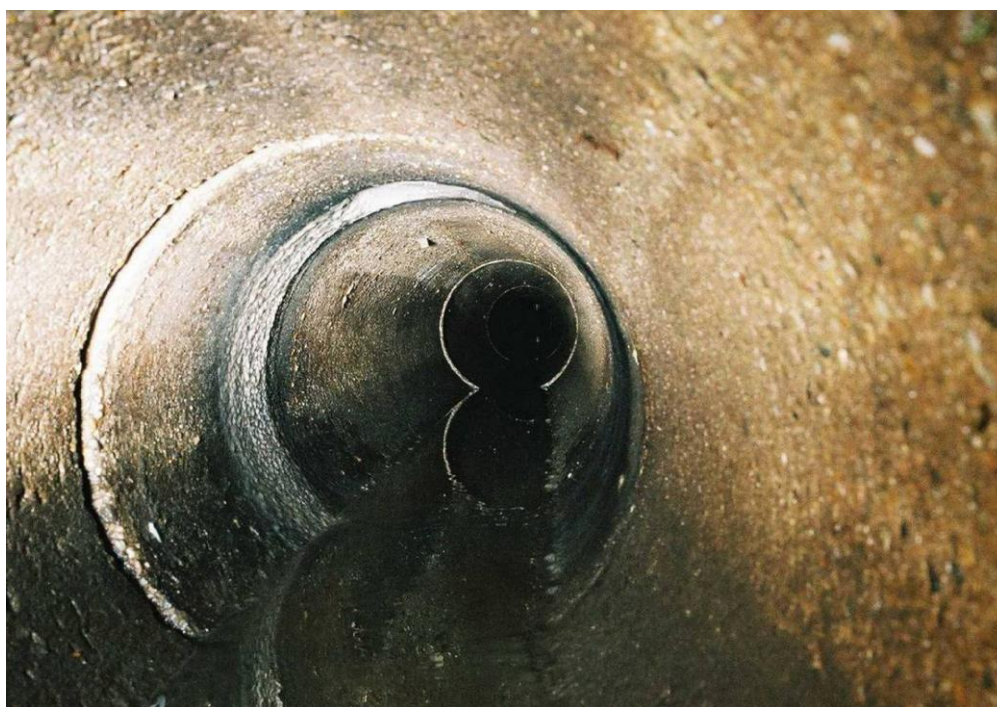
Figure F.26 — Example of displaced joint (radial)
