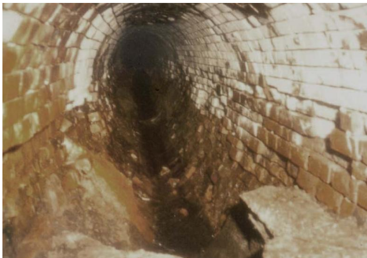
Figure F.16 — Example of missing mortar
