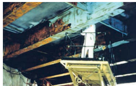
Fig. 40 Sodium-hydroxide-base chemical stripper applied to underside of bridge deck
