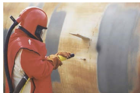
Fig. 24 Open-nozzle abrasive blast cleaning. Photo used with permission from SSPC: The Society for Protective Coatings
