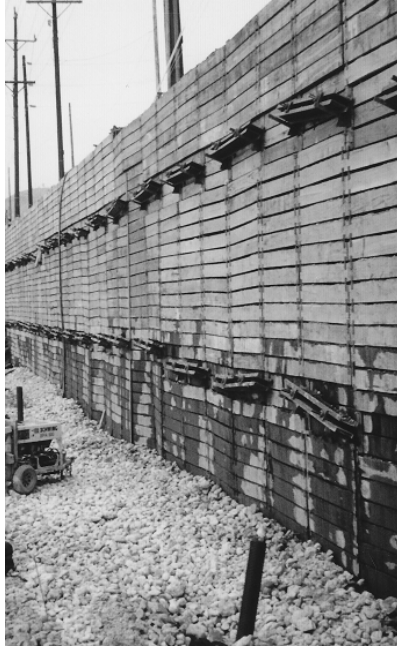
FIG. 2. Driven soldier beams with walers
