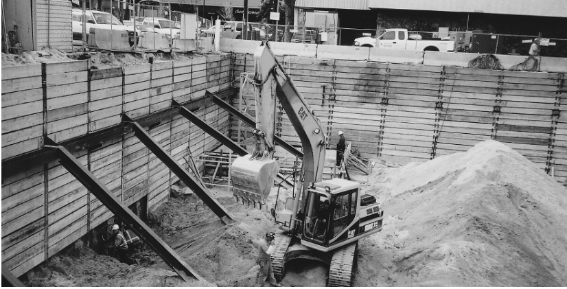
FIG. 1. Internal bracing and wale, left wall. Tiebacks, right wall, Denver, CO
