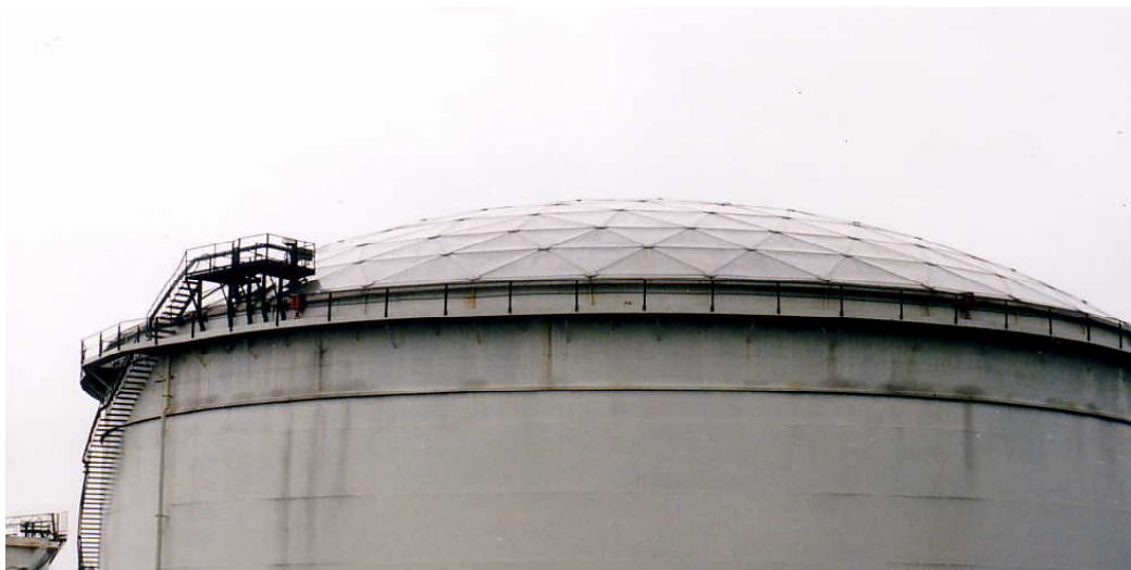
Photograph 3 Geodesic tank roof at an overseas refinery
