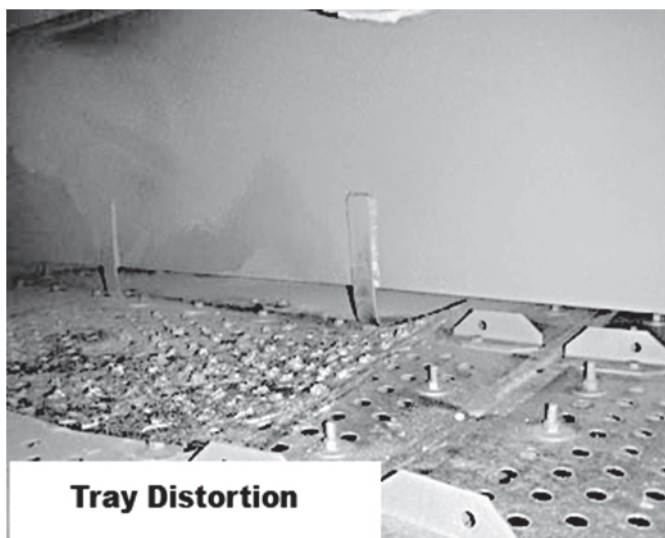
Figure B.9—Sieve Tray Distortion
