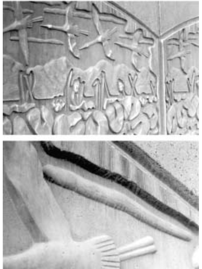
Fig. 1.1(c)—Close-ups of surfaces resulting from good consolidation.
