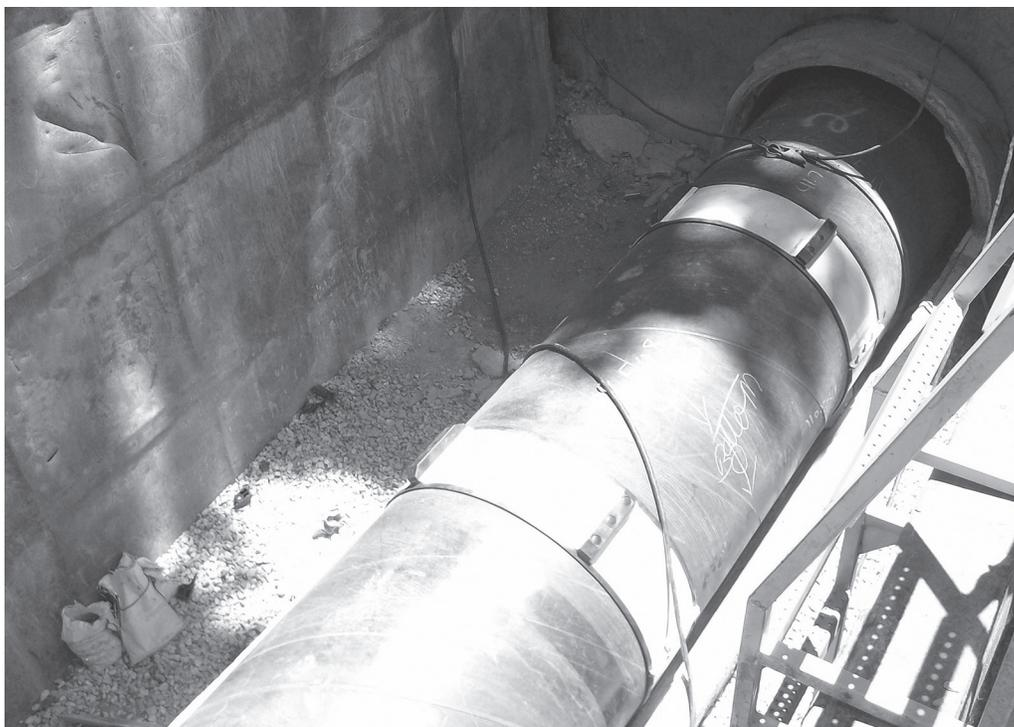
Figure 12-4 Steel slipliner section being inserted into host pipe with casing spacers
