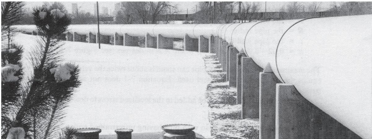
Figure 9-2 Saddle supports for 78-in. pipe
