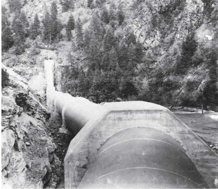
Figure 9-7 Ring girders on 111-in. pipe
