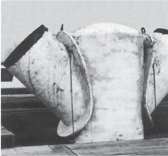
A single curved plate serves as reinforcement for each branch of this 96-in. × 66-in., 90° included angle wye.
