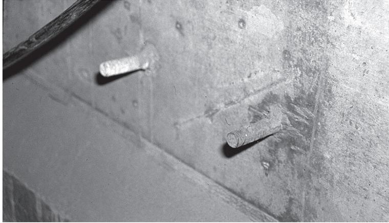
Figure 10-8 Corroding anchor bolt contacting reinforcement is subject to differential pH corrosion in water holding basin
