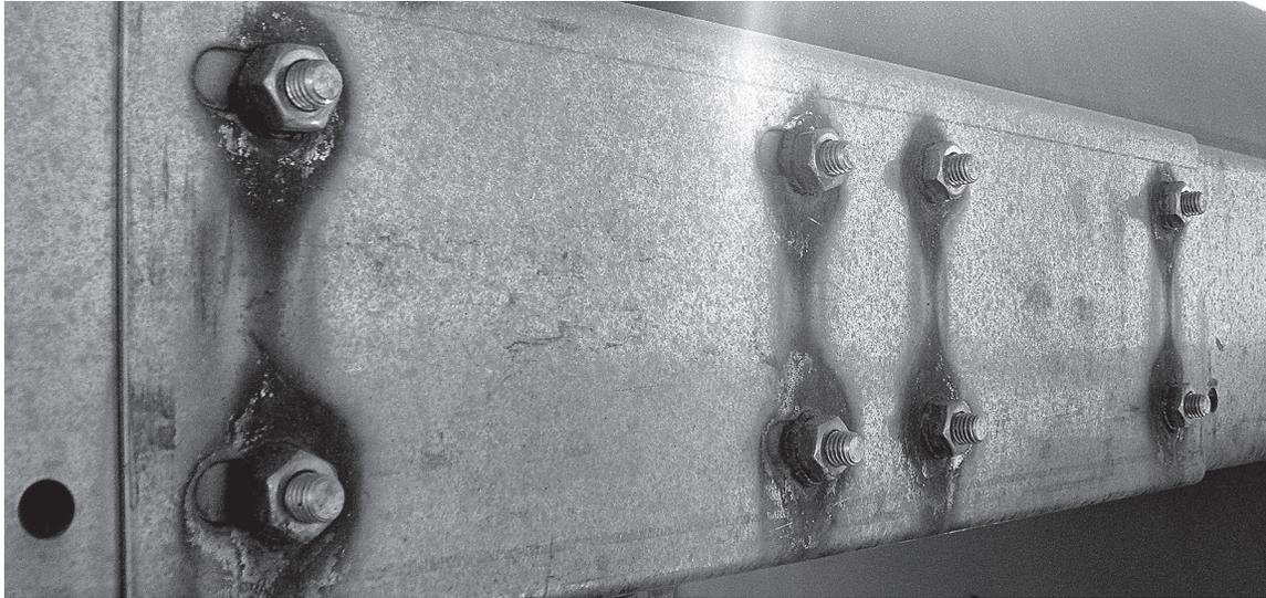
Figure 10-3 Dissimilar metal corrosion between stainless-steel base metal and carbon steel fasteners
