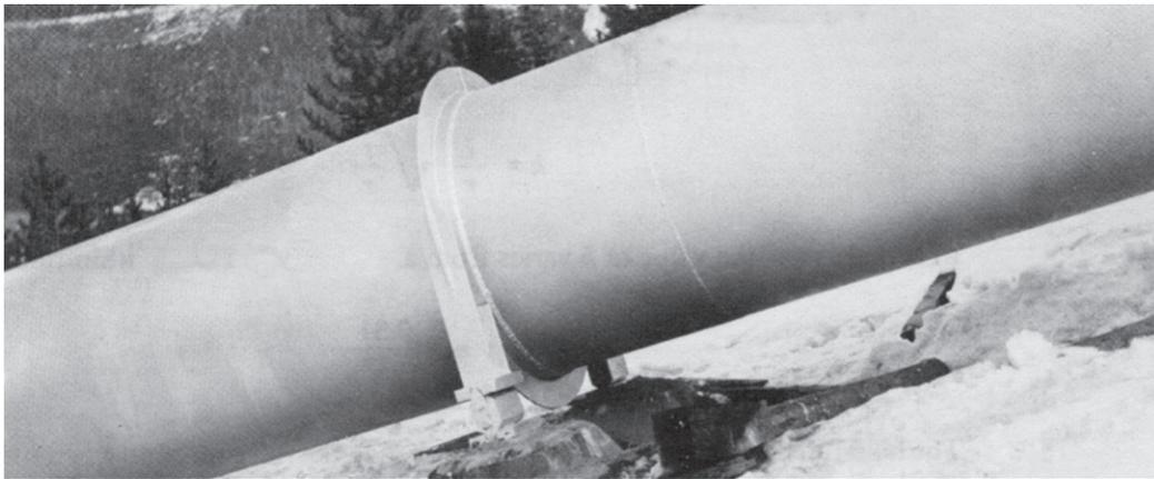
Figure 9-3 Ring girders provide support for 54-in.-diameter pipe
