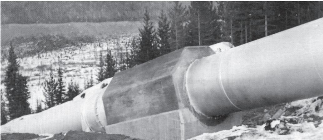
This block anchors a 66-in.-diameter pipe against longitudinal movement.
