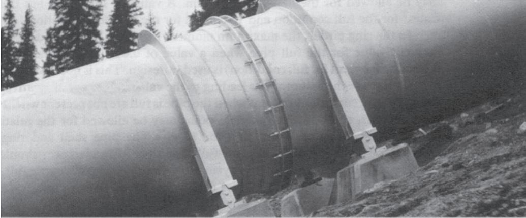
The rings are supporting a 54-in.-diameter pipe laid on a slope.
